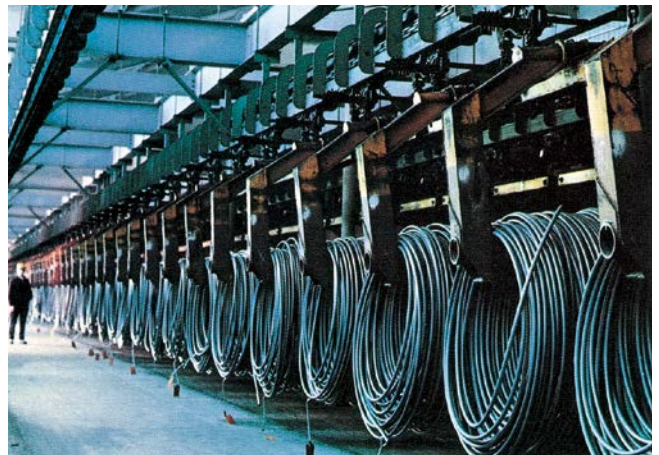
Power & free conveyor system
