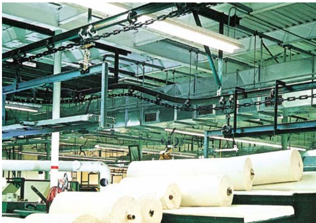
Trolley conveyor system
