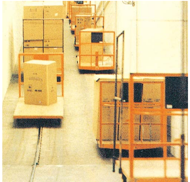
Towline conveyor system for carton transport
